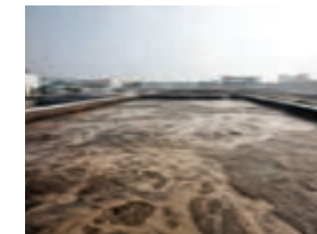
Named the Leader in Wastewater Treatment for Chemical Industrial Parks by ChinaWaterNet at the China Water Industry Annual Award 2013
