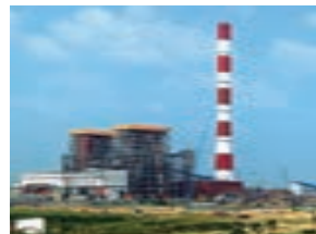
Marked a milestone at our first power project in India, Thermal Powertech Corporation India, with the synchronisation of the plant's first 660-megawatt unit to the grid
