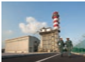
Commenced operation of the 400-megawatt Sembcorp Cogen @ Banyan in October, strengthening our market leadership on Jurong Island, Singapore
