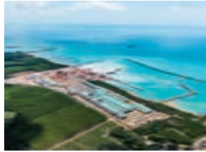
Estaleiro Jurong Aracruz commenced initial operation in the second half of 2014. The yard also received its first drillship unit, Arpoador
